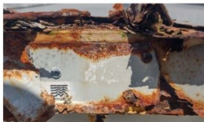
Coated roof edges prior to replacement
