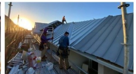
During Tedlar® roofing installation
